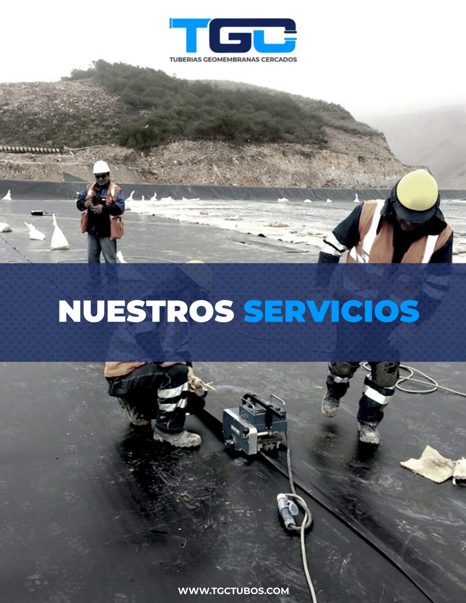
A construction site showing workers in safety gear (hard hats, high-visibility vests) working on a large-scale geomembrane liner. One worker in the foreground is using a specialized welding machine to join sheets of the liner. Another worker in the background is holding a device, possibly a surveying instrument. The site is outdoors, with a rocky hillside in the background and a body of water or a large excavation area in the foreground.
